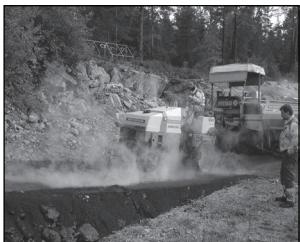
The heating cable(s) can be covered in asphalt with a maximum temperature of 160 °C.
