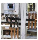
IBS Flat Insulated Braided Conductors are the ideal ready-to-install flexible wire replacement solution. They connect directly to the front access terminals of an electrical device without the need for additional accessories, such as angular connectors, spreaders, ring terminal connectors or extenders. IBS Flat Insulated Braided Conductors are available in cross section of 25 and 50 mm $^2$  (49.34 and 98.68 kcmil), lengths from 165 to 1,130 mm, and amperages ranging from 177 to 274 A.
