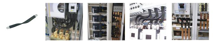
IBS Flat Insulated Braided Conductors are the ideal ready-to-install flexible wire replacement solution. They connect directly to the front access terminals of an electrical device without the need for additional accessories, such as angular connectors, spreaders, ring terminal connectors or extenders. IBS Flat Insulated Braided Conductors are available in cross section of 25 and 50 mm<sup>2</sup> (49.34 and 98.68 kcmil), lengths from 165 to 1,130 mm, and amperages ranging from 177 to 274 A.
