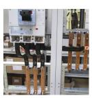
IBS Flat Insulated Braided Conductors are the ideal ready-to-install flexible wire replacement solution. They connect directly to the front access terminals of an electrical device without the need for additional accessories, such as angular connectors, spreaders, ring terminal connectors or extenders. IBS Flat Insulated Braided Conductors are available in cross section of 25 and 50 mm² (49.34 and 98.68 kcmil), lengths from 165 to 1,130 mm, and amperages ranging from 177 to 274 A.
