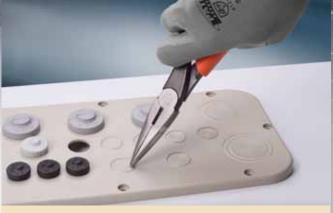
Make appropriate size hole to blind plate or knock-out plate. Avoid rough and sharp edges.
